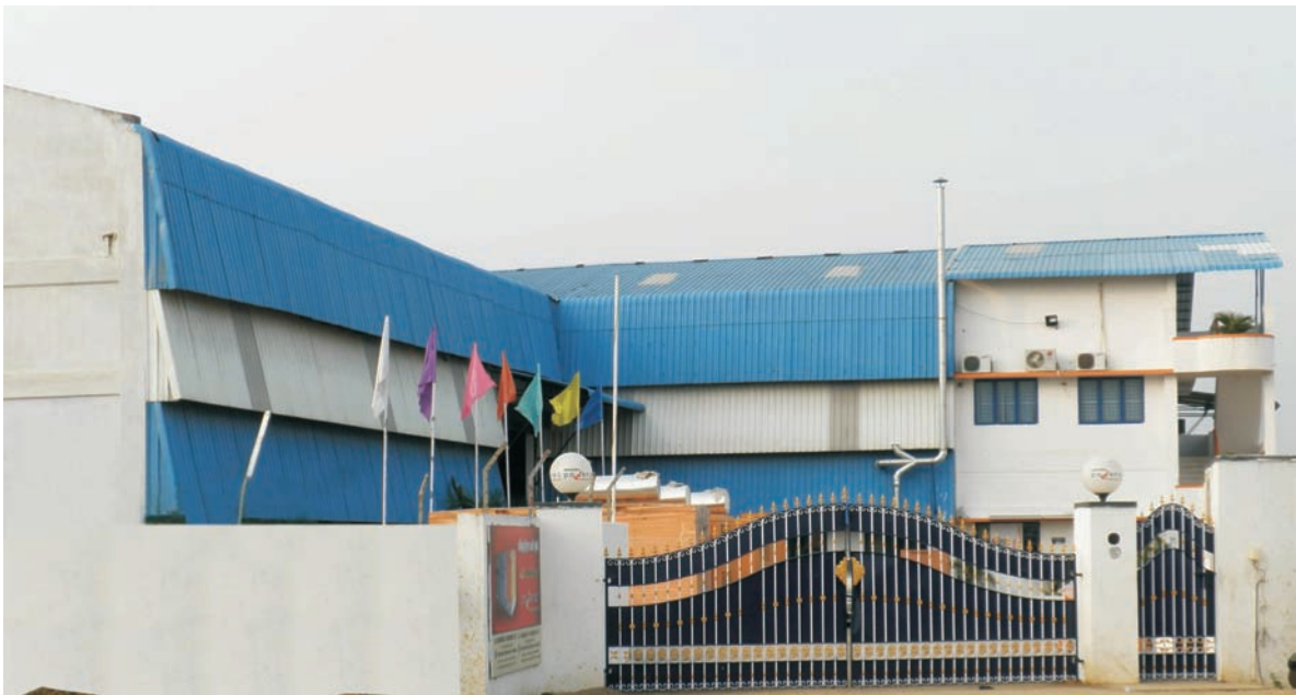
SIAS - Padappai facility (located in growing industrial area )
